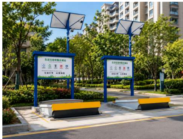
Roadside installation with solar monitoring kiosk — suited to small front-end collection vehicles using market-standard rear-loading compactor trucks
